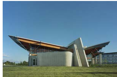
Heifer International Education Center Little Rock, AR Polk Stanley Wilcox Architects
