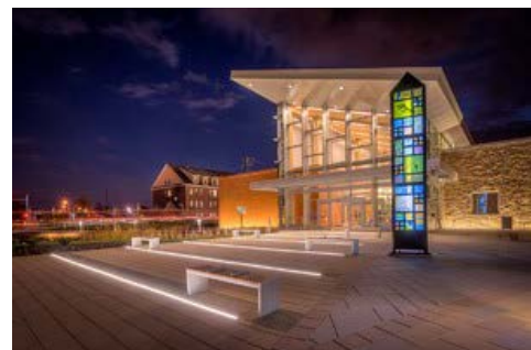
Laurel Branch Library Laurel, MD Grimm+Parker Architects
